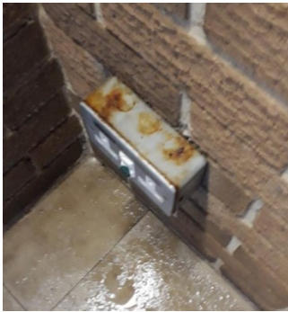
< Condense dropping on outlets not IP rated.
