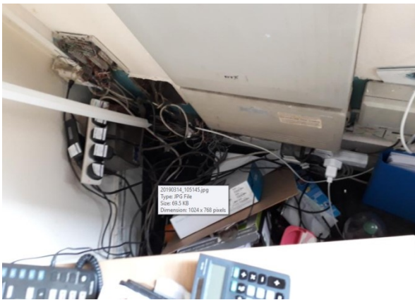
< Condense dropping on outlets not IP rated.
